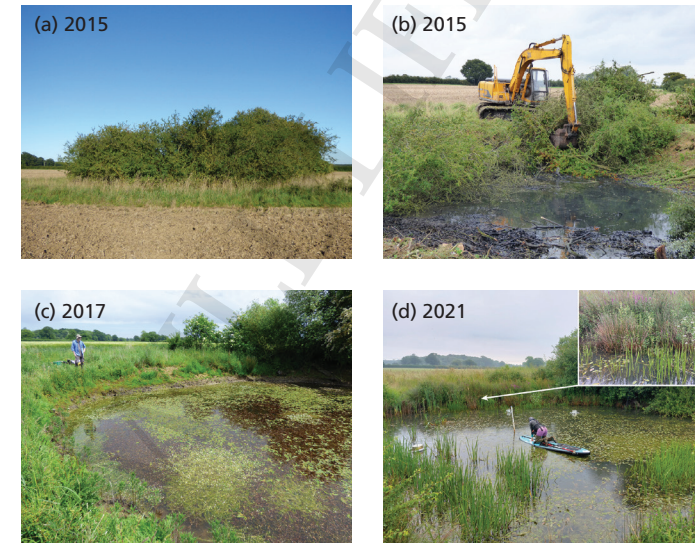
Figure 3. A mid-arable Norfolk pond before (a), during (b) and two (c) and six (d) years following restoration via major scrub and mud removal by the Norfolk Ponds Project. Carl Sayer
